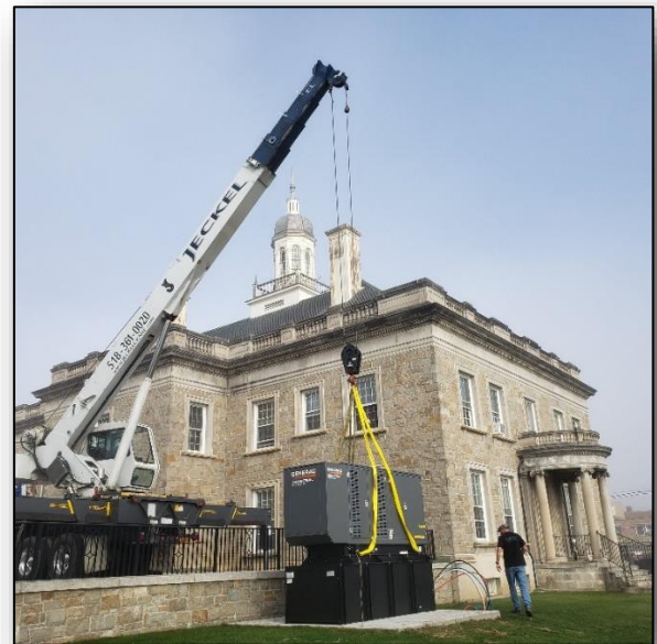
Generator is lifted into position.
