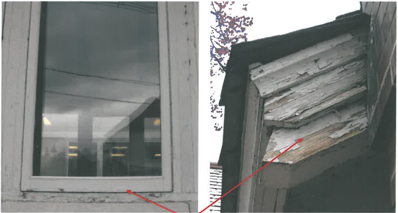
Scrape, caulk, and repaint peeling soffit and window areas
